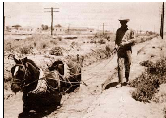
Figure 1. Dredging a canal in the Salt River Valley, circa 1900. Photo courtesy of SRP.
