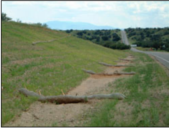
Bank Stabilization and Erosion Control along a highway (Photo: Lainie Levick)
