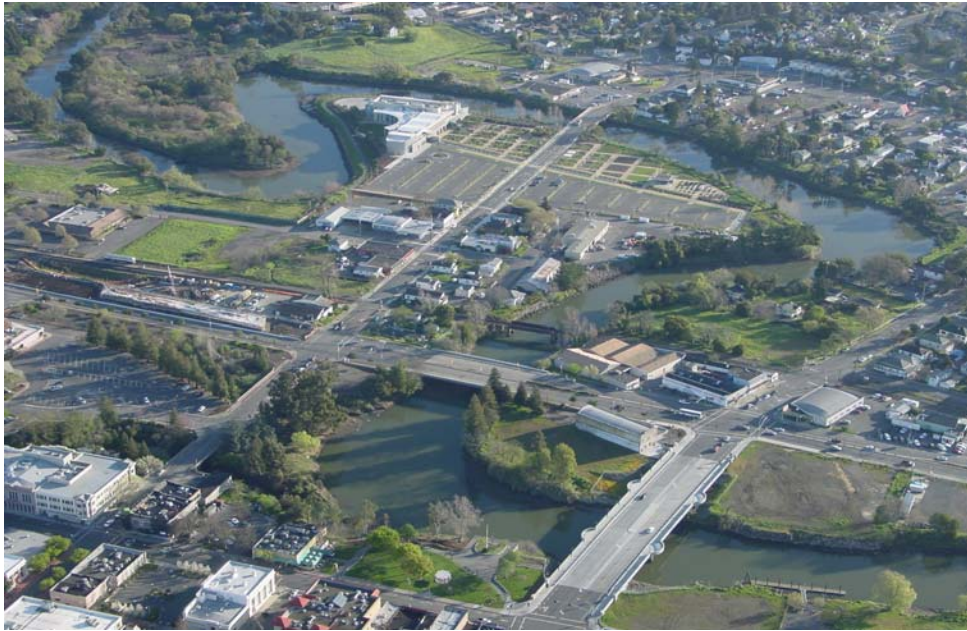
Figure 9. The Napa River at the oxbow in downtown Napa, before construction of the dry by-pass channel.
