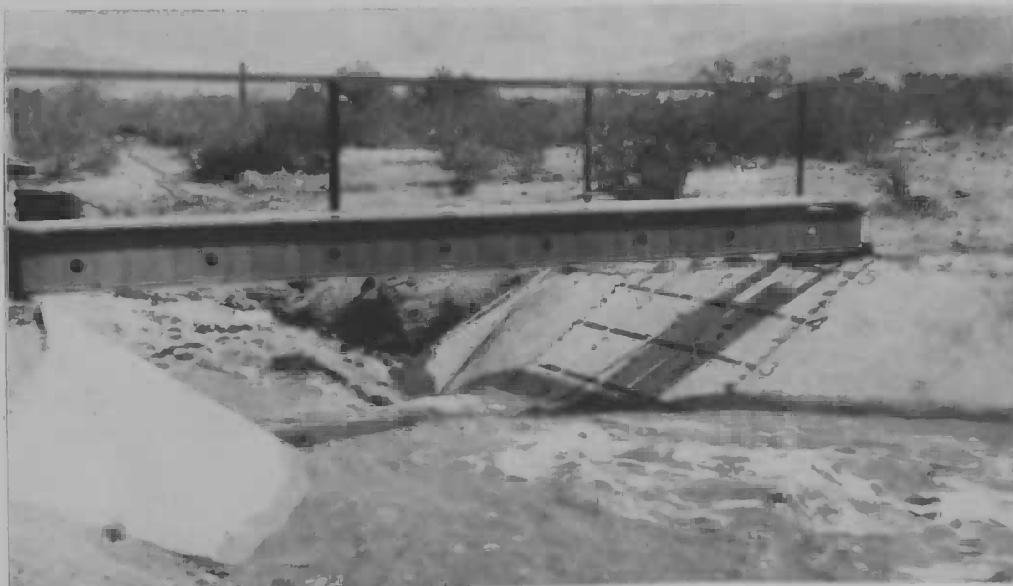
FIGURE 3.10 FLOW CONDITIONS--FLUME NUMBER 1
