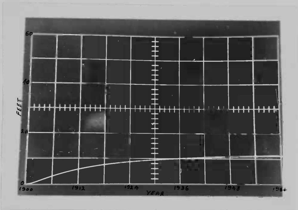
Fig. 25c.--Hydrograph Showing Very Little Rise In Ground-Water Level Due to Location Near the River - Analog Model.
