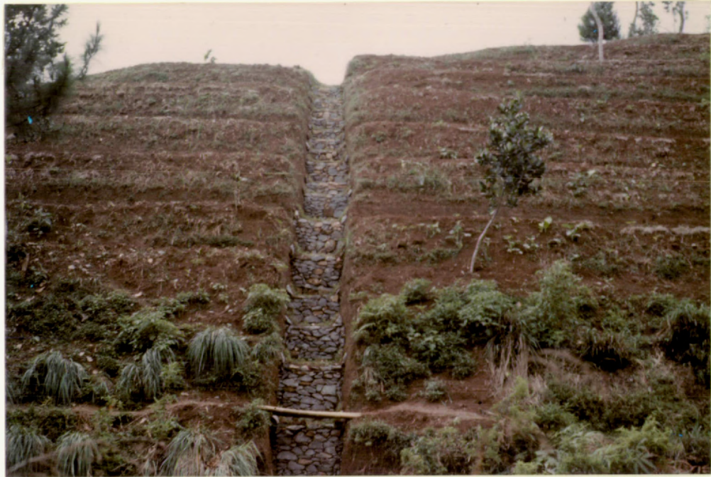
Figure 6. Waterway built across the contour line
