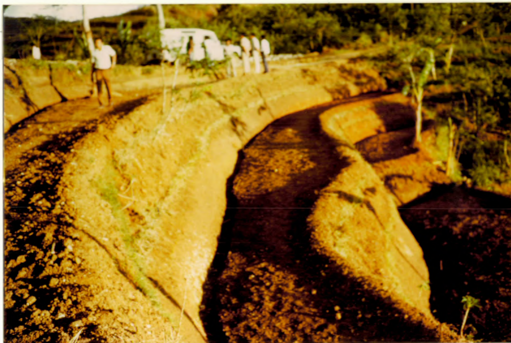
Figure 10. Grass plantation on risers of new terraces
