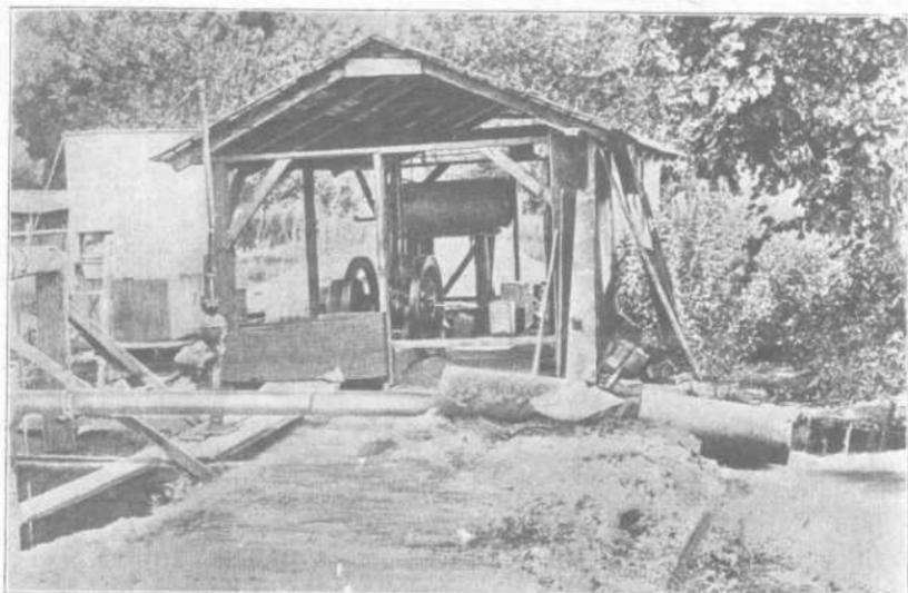
Small gasoline engine raising Santa Cruz underflow for irrigation.
