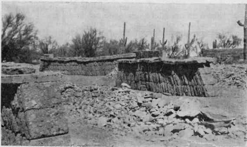
Plate II.—Adobes made of Pinal gravelly stony loam from which coarse aggregate has been screened out. Note that a large part of the waste consists of grayish white chunks of the caliche hardpan. This material represents about the extreme in coarse aggregate which may be used in making adobe. Lot 10 of the test adobes was made from this material, but more of the coarse aggregate was removed than in the case of those shown above.
