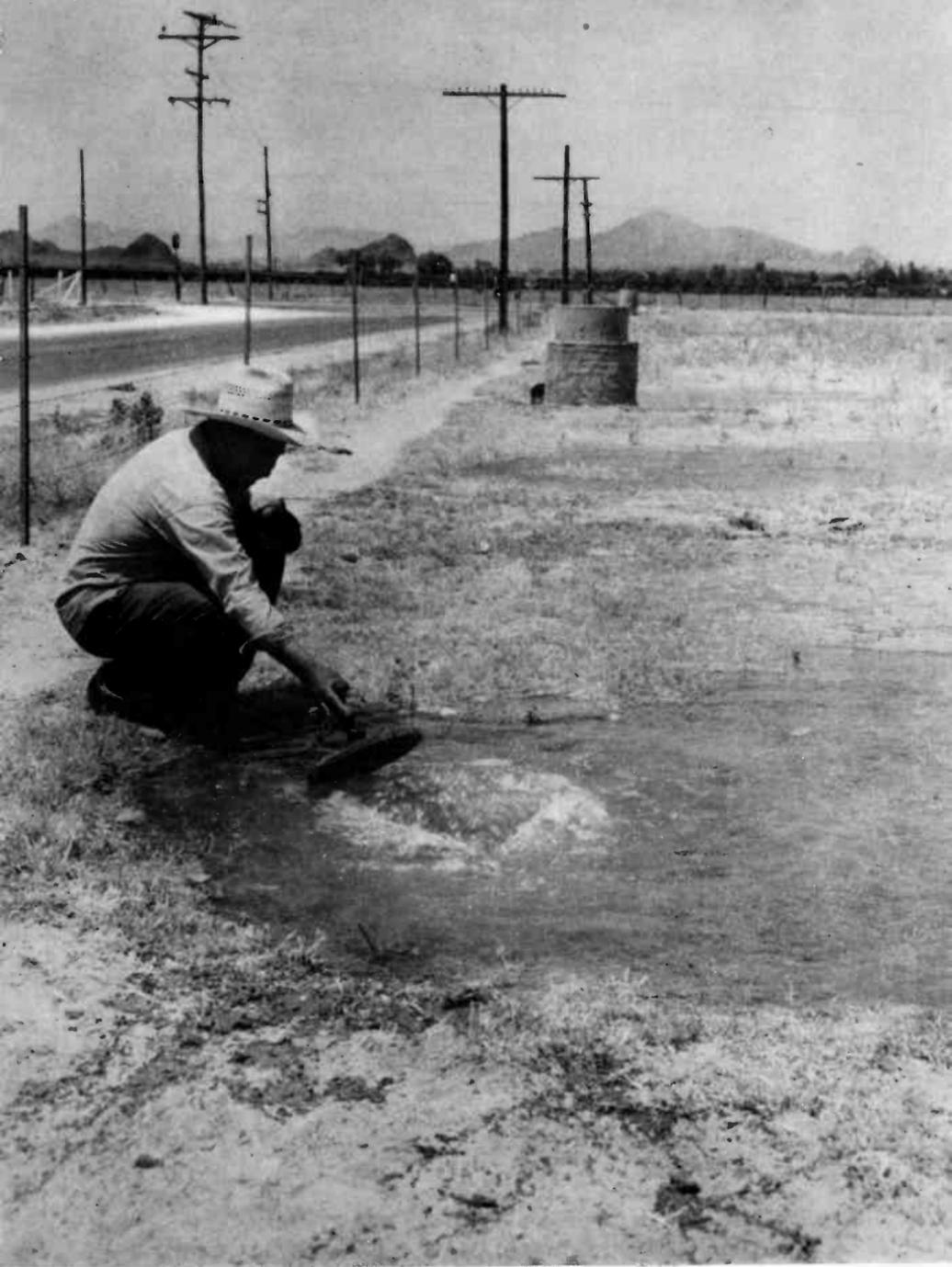
PLATE IV.—The Underground Pipe System. The entire system is underground except for the standpipes and the irrigation valves.
