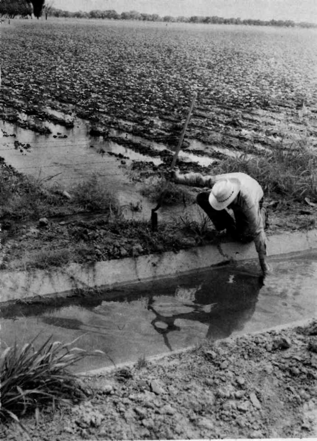
PLATE III.—The Concrete-lined Ditch. The concrete lining reduces the amount of water lost through seepage.
