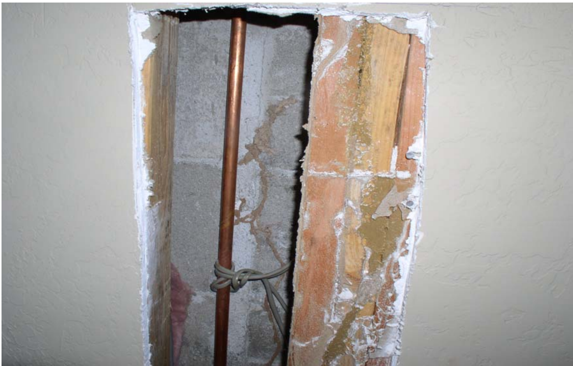
b) Exposed wall showing termite trails where Pestfinder detected motion.
