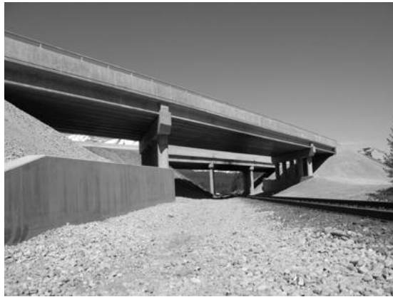
(a) Highway Bridge with Bents Consisting of Exposed Cap Beams and Five Piers
