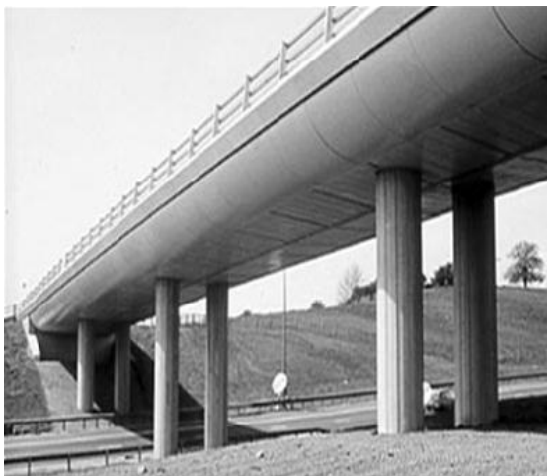
(b) Highway Bridge with Bents Consisting of Hidden Cap Beams and Two Piers
