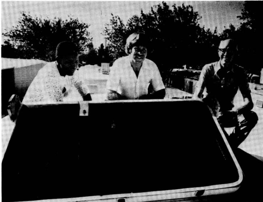
M. Nikyema, left, and his interpreter G.B. Plotkin, center, examine simple solar energy supply system using a junked refrigerator door fitted with coils and copper tubing under the heavy glass top, as a solar hot water heater. Owner and designer Gilmore Gilbertson, Tucson, right.
