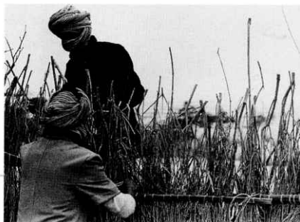
In Mauritania, project participants build windbreaks to retard desert encroachment.
