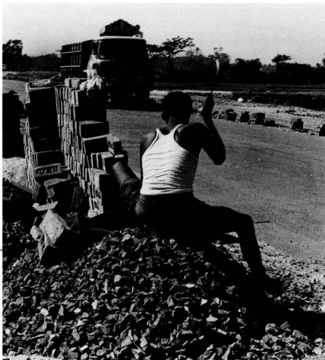
In Bangladesh, building roads provides employment and improves rural communication.
