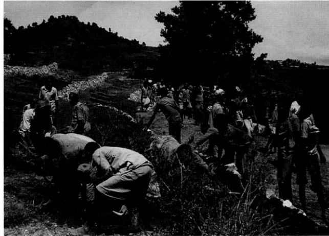
Ethiopian farmers and their families dig terraces and build stone walls, thus strengthening the agricultural infrastructure, in return for food aid.
