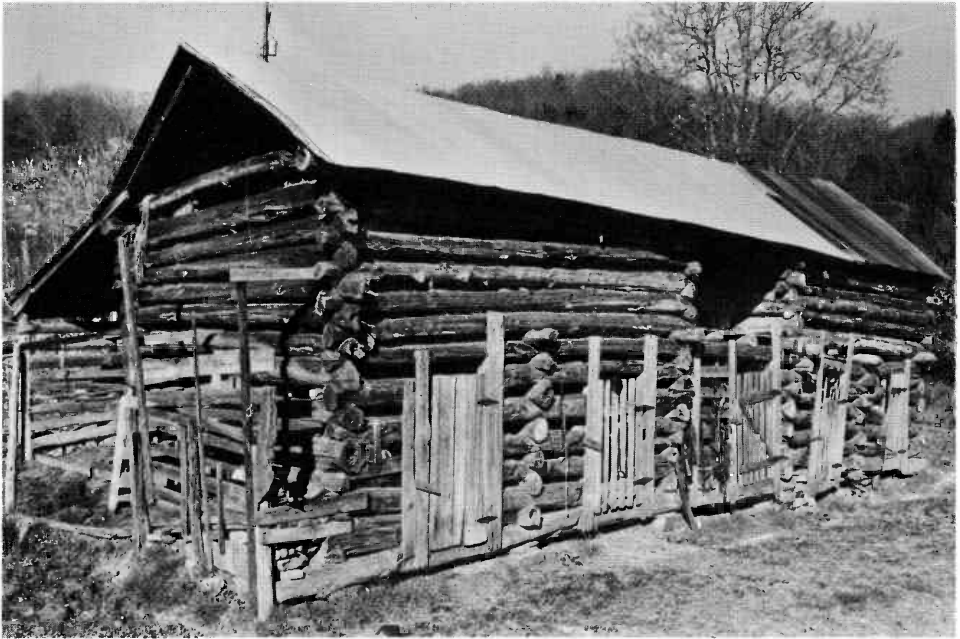
Figure 1. A large collection of eastern red cedar logs in the Lancaster Barn. Six cutting dates between 1854 and 1867 indicate that this barn was built in part with re-used timbers following the Civil War.
