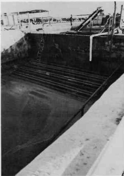
Heat-transfer pipes warm the manure mixture with heat from the bio-gas-fueled engine. The higher temperature speeds bacterial action.
