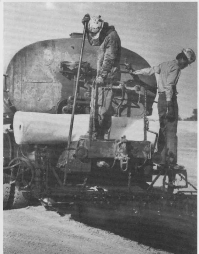
**Crew member Robert Curlyhair (right) and UA graduate student Ken Vogler help with treatment of the catchment slope to increase runoff. White fiberglass gauze was unrolled from the back of the truck, then sprayed with hot asphalt.**
