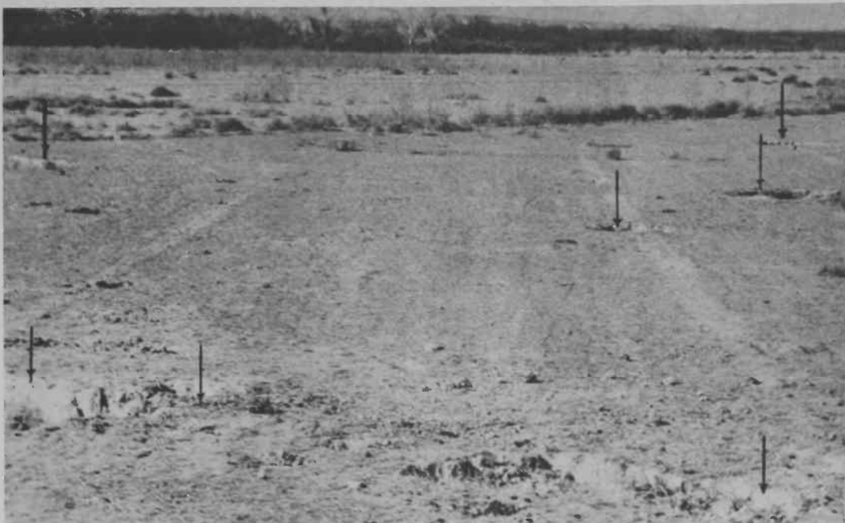
↑ Pipe entrances in an alfalfa field near Pomerene. The arrows point at the holes where the soil has caved into the underground tunnels. SCS Photo.
