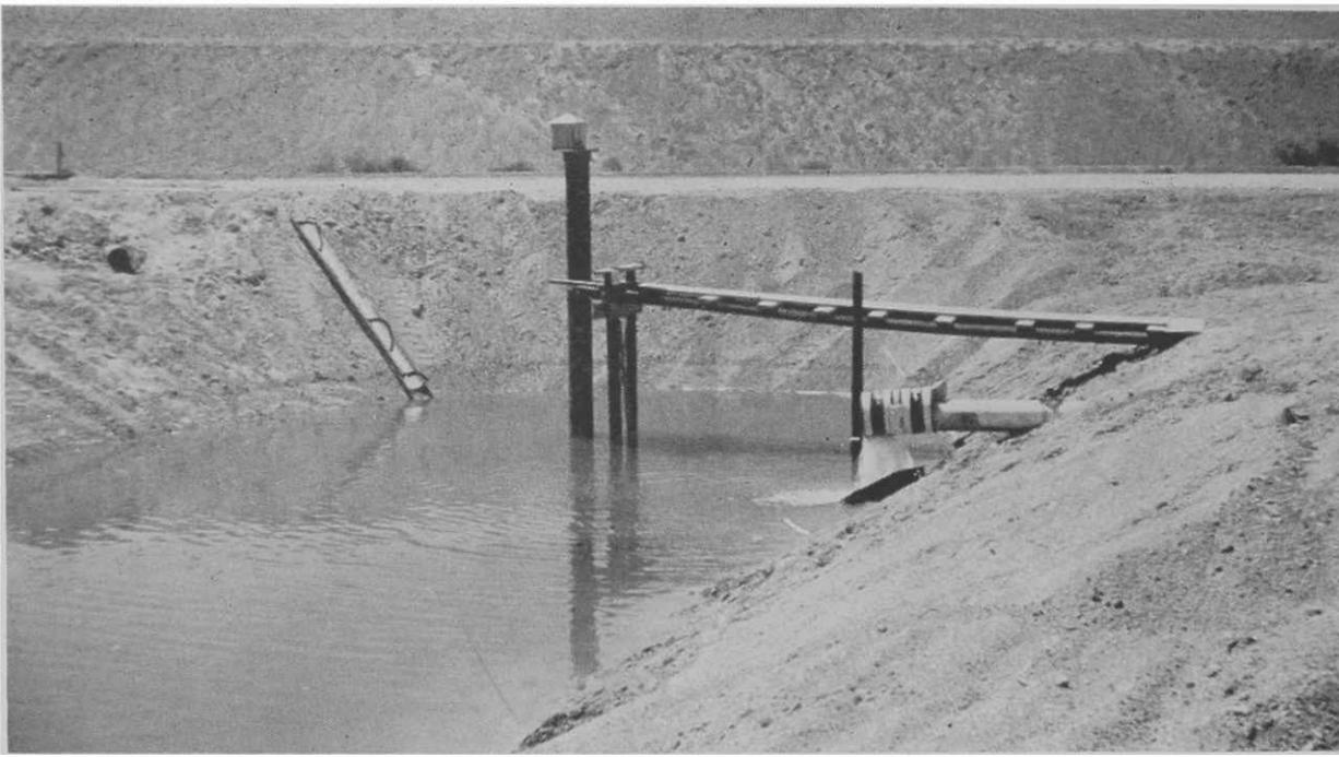
AT LEFT, VIEW of the Beardsley recharge pit, showing the flood control dam in the background. Walkway leads to a water level recording device installed in the vertical standpipe.
