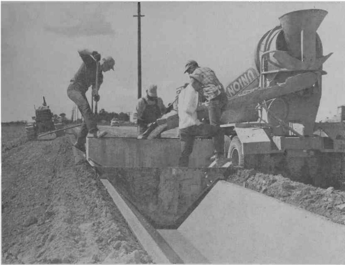
**THIS CONCRETE DITCH** lining machine, invented in Phoenix, is just one of many things developed to increase the efficiency of agriculture in the Salt River Valley.
