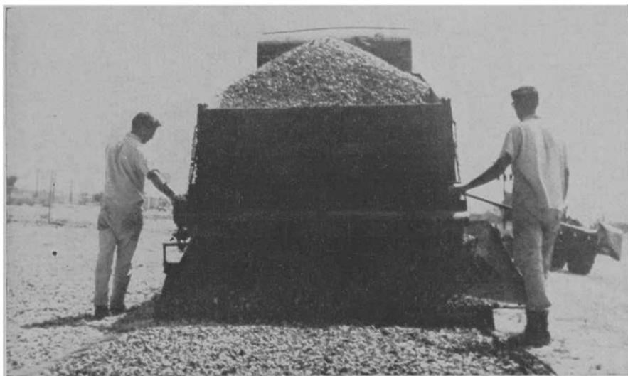
**LAYING PLASTIC** and covering it with gravel in one operation.
