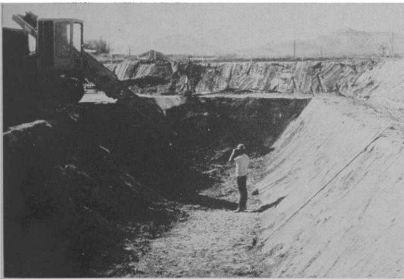
EXCAVATING STORAGE tank with Gradall.
