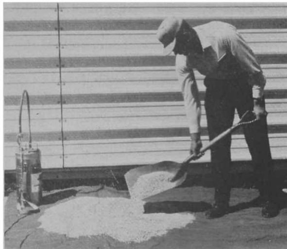
SAND DROPSEED and rice hulls being dry mixed before application of methyl cellulose sticker solution. Mixing is done with scoop shovel on canvas tarp. Pressure sprayer for applying sticker is at left.
