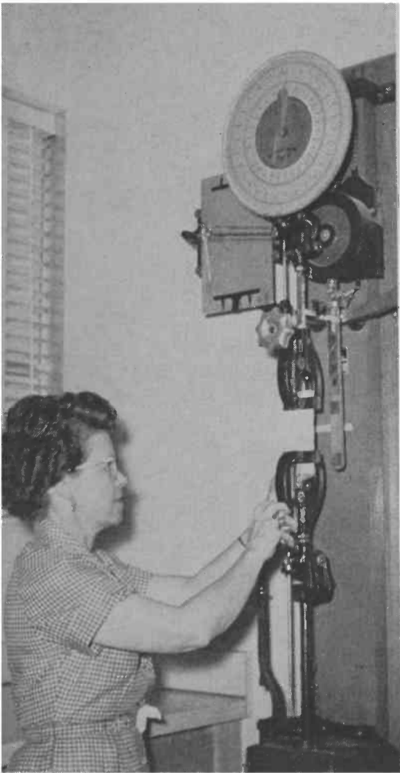
TESTING TENSILE STRENGTH of cotton fibers is Miss Ruth Allen, chairman of the Division of Clothing, Textiles and Related Arts.
