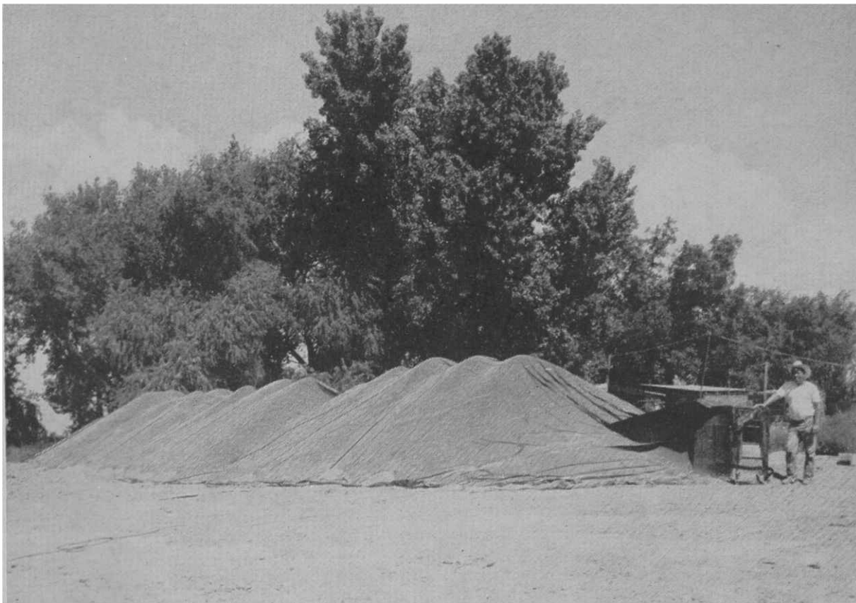
SUCTION-CONTROLLED plastic temporary grain storage setup in actual use in Arizona. Notice how effectively the suction causes the plastic to cling to the contours of the piles of grain. Also note crimped edges of the plastic, where it meets the ground.
