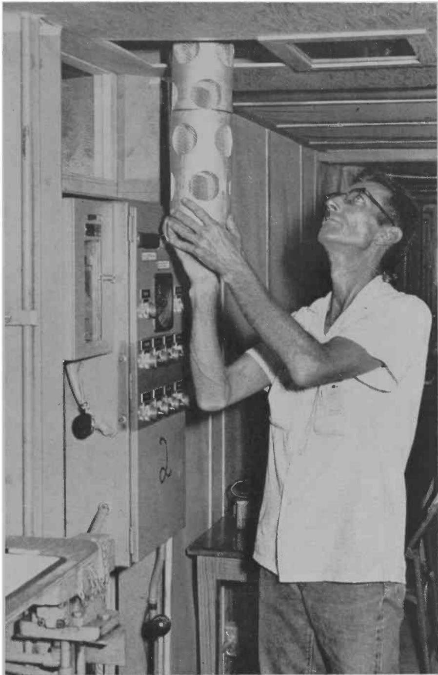
**AFTER LARVAE HAVE** pupated, about 31,500 are placed in each canister, the canisters then automatically carried into a Cobalt-60 chamber, where the screwworm flies are sexually sterilized by exposure to gamma rays. The remote control mechanism, lead shields and constant checking protect persons working on this project as well as other persons in the vicinity.
