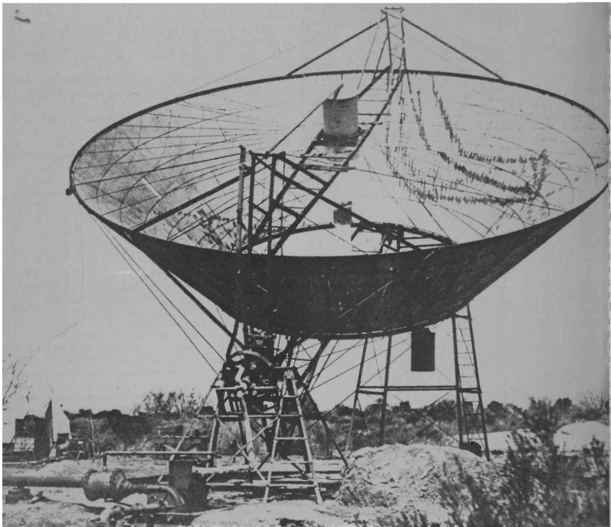
*SHORTLY AFTER the turn of the century, this solar power plant was pumping irrigation water near Phoenix. The conical collector was 33 feet in diameter.*
