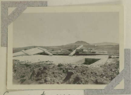
Cement cover over underground Cistern.
