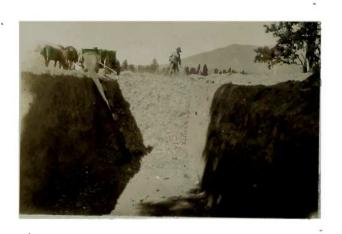
Filling the trench sile of the mountain Dairy. The soil, cinuary in nature and well-arained, is almost ideal for preservation of silage. More siles, of cheap construction are needed in this county.
