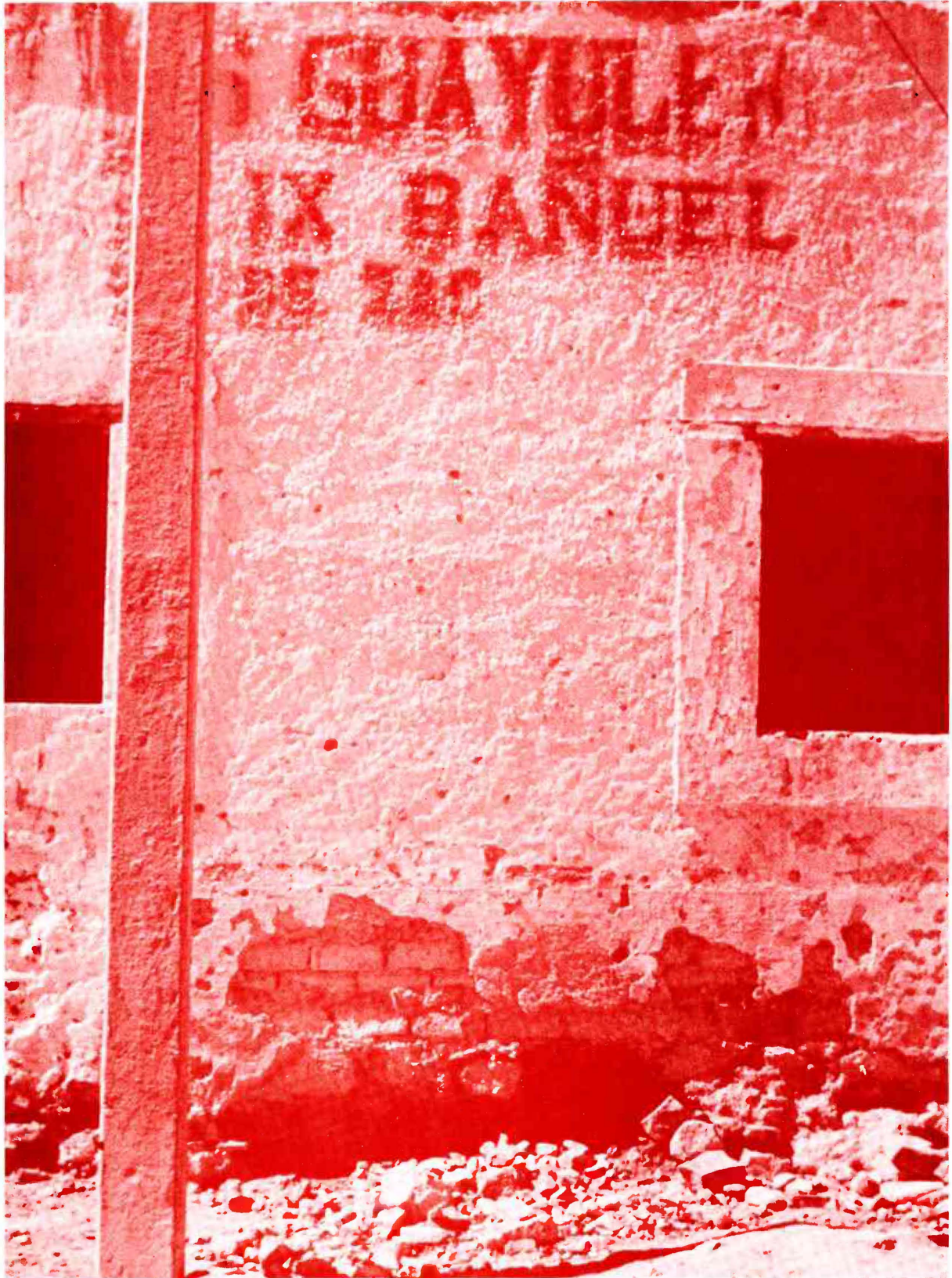
Ruins of old Guayule processing plant, Cedros, Zacatecas
