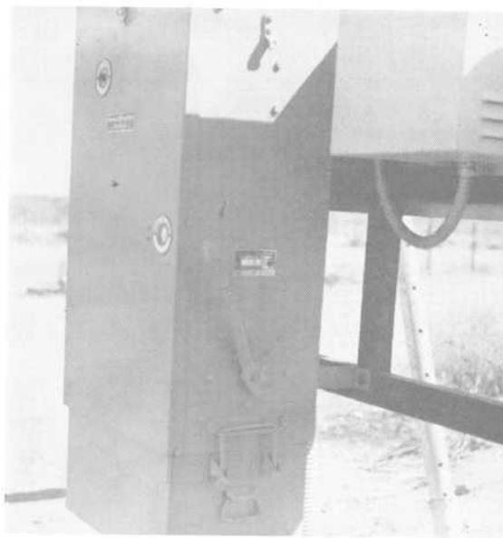
**Overload protection** devices are often installed inside the motor controller cabinet although they may be mounted in a separate location. Their purpose is to interrupt the circuit before the motor windings become hot enough to cause damage to the insulation. The devices must be so constructed that the circuit is not broken by the high starting current but is broken as a result of prolonged currents only slightly greater than the normal running current.
