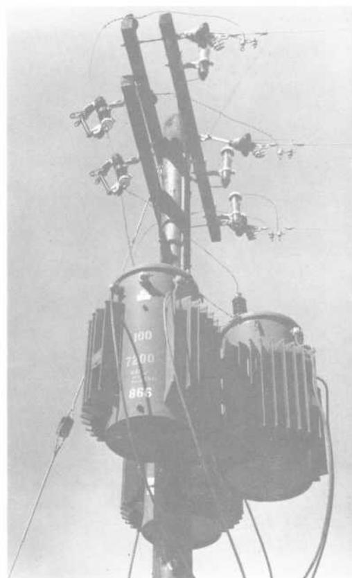
**A main switch or circuit breaker** is needed unless the oil-filled switch and circuit breaker is used in the primary circuit or a factory-built pump panel containing a switch is used in the secondary circuit. In this way, a means is provided for disconnecting equipment so tests and repairs may be made.
