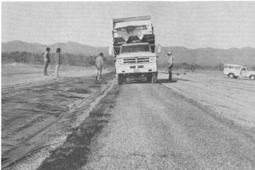
FIGURE 4. CONSTRUCTION OF APAC CATCHMENT IN PROGRESS AT SELLS, ARIZONA
