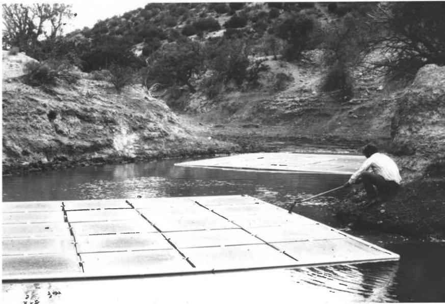
FIGURE 9. ASPHALT CHIPCOATED COUPLED EXPANDED POLYSTYRENE RAFTS ON A TYPICAL EARTH STOCK TANK.
