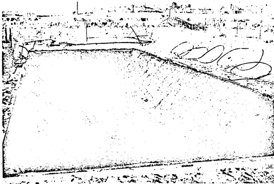
FIGURE 16. ASPHALT-RUBBER LINING INSTALLATION
