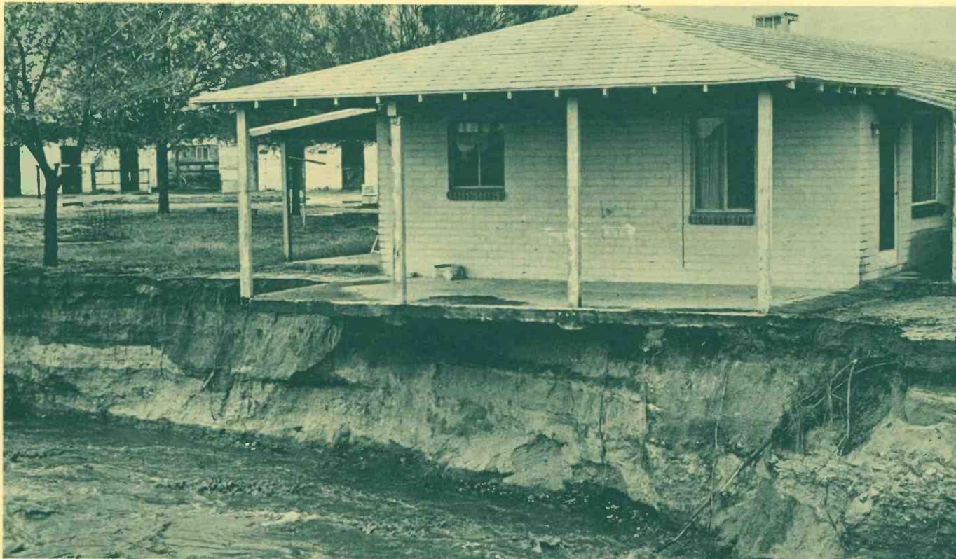
Floodwaters in southern Arizona, sometimes of high velocity and with a high concentration of runoff, scour stream channels that then could shift and change. Severe property damage may result. *Photo: Fred Wehrman*
