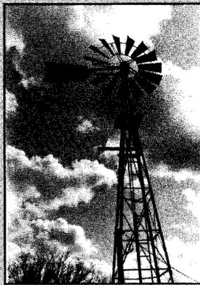
*The windmill is a low-tech device for bringing groundwater to the surface.*
