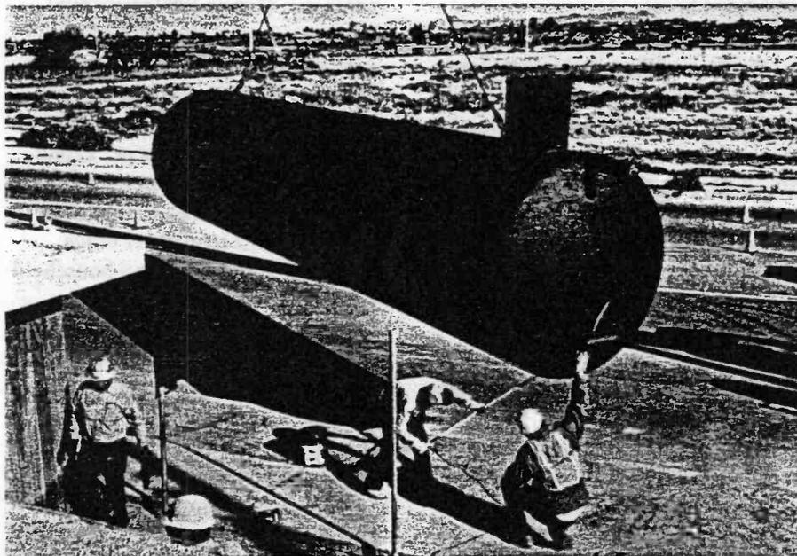
*A tank to store graywater is installed at Casa del Agua, Tucson's water conservation house. The tank is about six and one half feet in diameter, 30 feet long, and holds about 7,000 gallons. (Photo: Rocky Brittain)*
