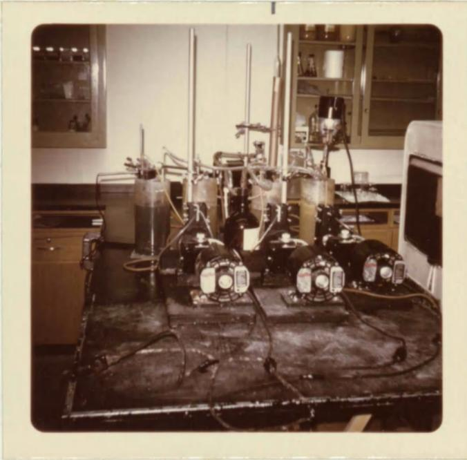
Figure 3.2 Phase one activated sludge reactors
