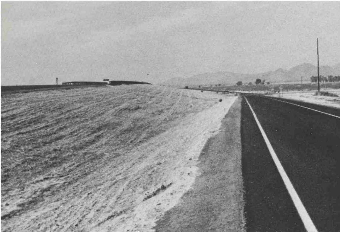
Figure 1. An area where two tons of hay per acre were anchored by crimping after having been seeded.
