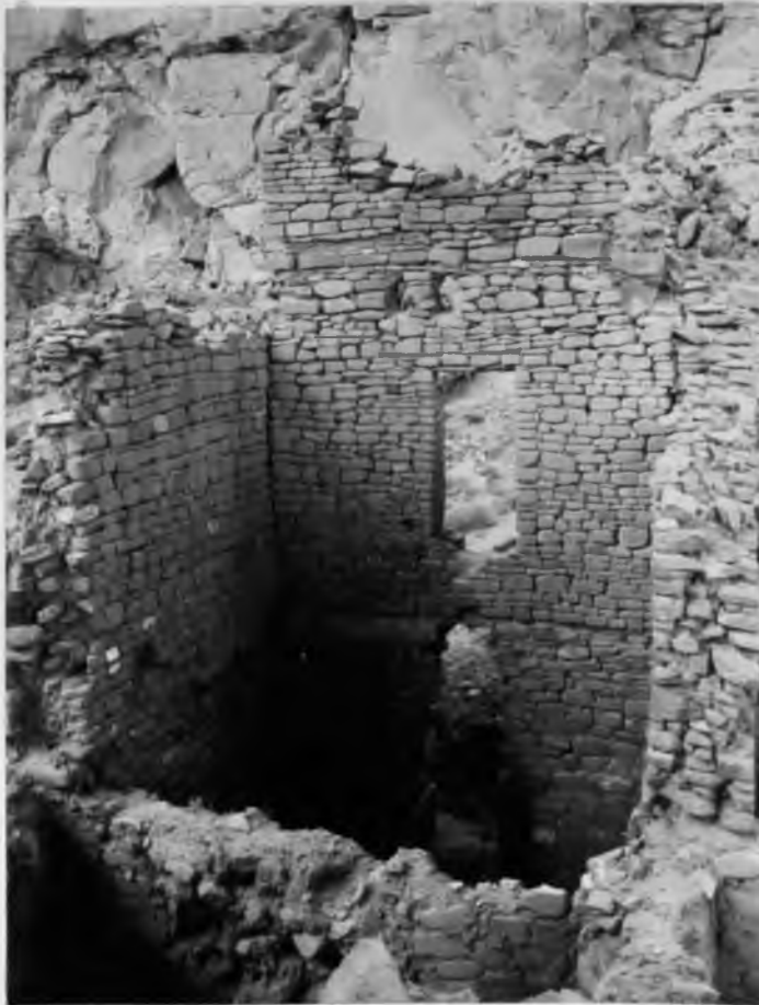
Plate IV. North wall of Room 11. Notice the three story construction. (Courtesy National Park Service)
