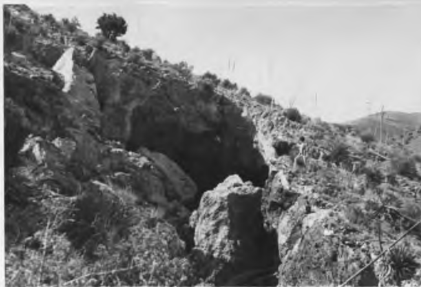
Figure 16. One of the many cavities on Queen Hill caused by the cave-in of underground workings.
