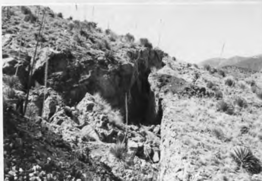
Figure 17. Small fault or fissure on Queen Hill caused by sub-surface slumping.
