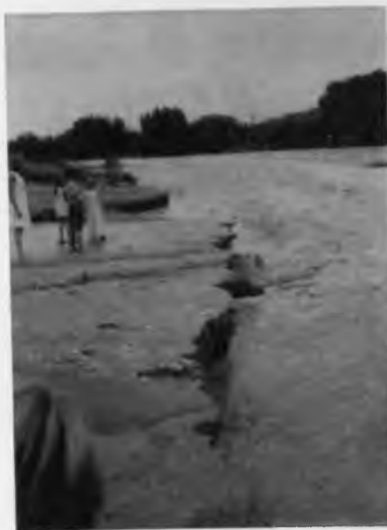
Figure 27. Bank Erosion during the Pantano Wash Flood. (Photo by R. D. Call)
