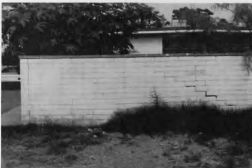
Figure 22. Wall Fracturing due to Collapsing Soils, North Fontana Avenue Just North of Grant Road.
