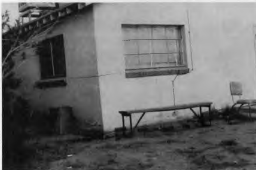
Figure 23. Building Fractures due to Collapsing Soils, North Fontana Avenue Just North of Grant Road.
