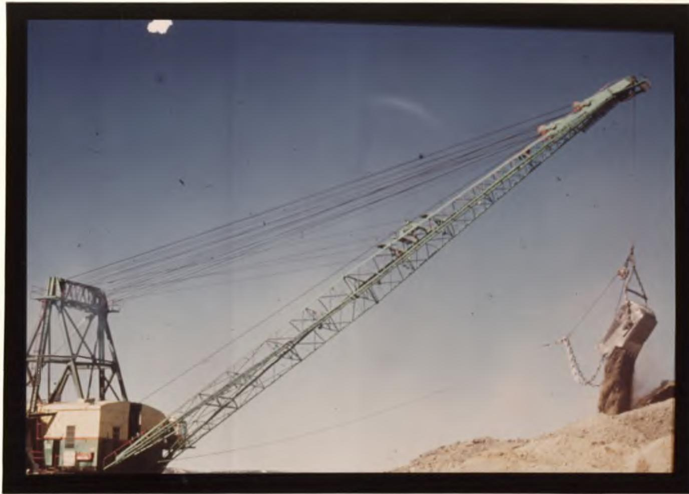
Figure 4. Peabody Coal Company dragline removing overburden to expose a coal seam. -- This huge machine removes the strata overlying the coal. The cab surrounding the engine and operator's controls is as large as a small house.
