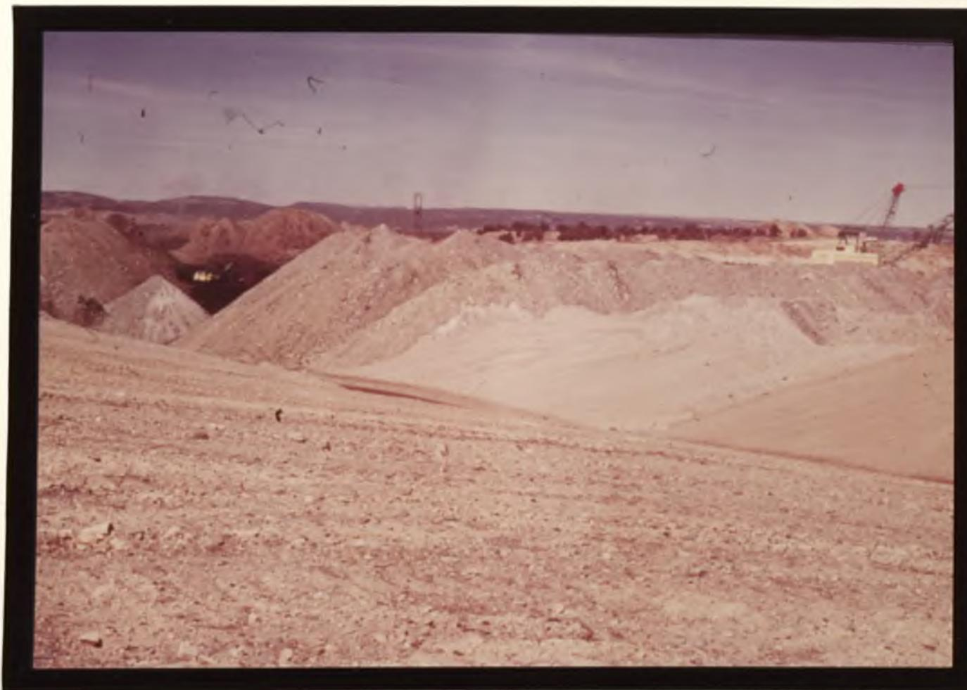
Figure 5. View illustrating recontoured and non-recontoured coal mining spoils banks. -- The foreground of this view depicts an area which has been leveled and recontoured. The steep-sided rows of spoil banks in the background show how the spoils look immediately after the coal is removed.
