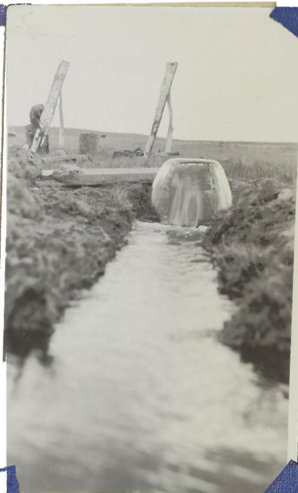
Well #9 of Joseph City Project Approx flow 160 Gals per min Reduced to 115 Gals per min when 90 other well drilled 100' East 1936
