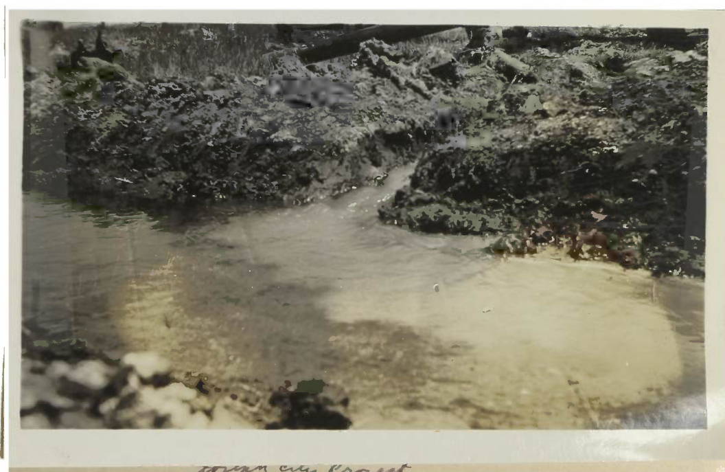
Flowing well Joseph City Project - V weir readings over period of 3 months average 130 gal per min. measured 190 gal p/m until other wells were drilled 1936
