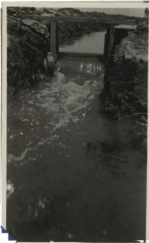
Wier measuring flow of all Flowing Wells of Joseph City Project Average 8 measurements July and August 750 Gals per Min. (8 wells) 1936
