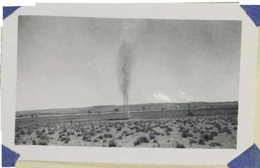
Blasting 100' well in Joseph City Project in effort to open water bearing, result - no increased flow resulted 1936
