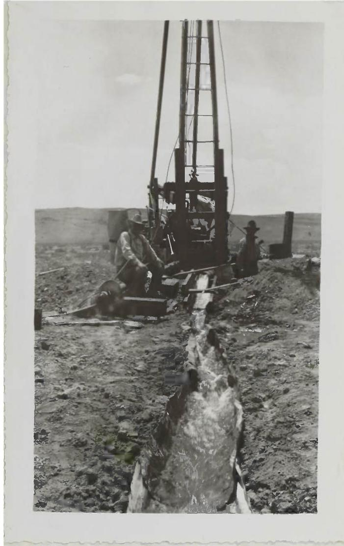
Fig. 1 Well at J. W. Rogers', Hunt, showing the water being pumped in this well which came within two feet of the top and was of high quality.
