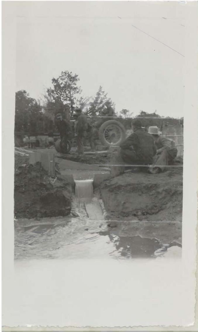
Fig. 14 Water at Harkey Well, Plenty, being measured by Weir, which produced 125 gallons per minute.
