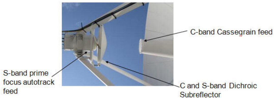
Figure 18 ViaSat Baseline L/S and C-band Dichroic Subreflector
