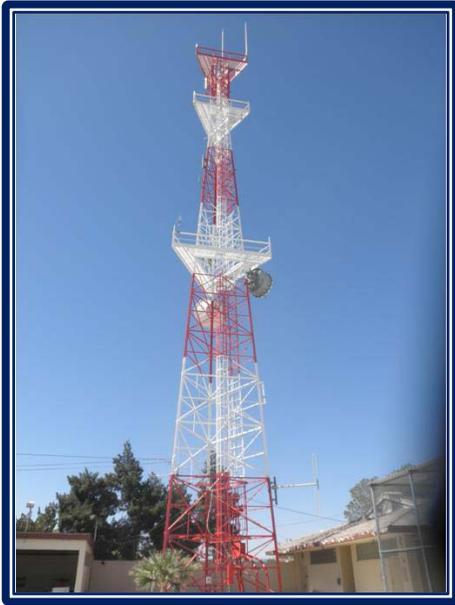
*Figure 12 – Ground Antenna System Mounted Atop a 180’ Tower*
