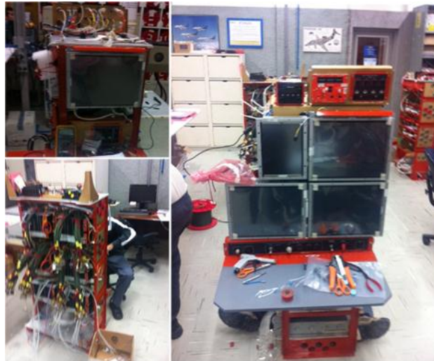
Figure 3: The FTI equipment is assembled in racks for rapid installation
