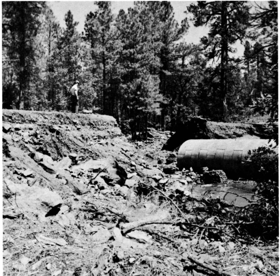
FIGURE 16. DAMAGE TO FOREST ROAD ON THE COCONINO NATIONAL FOREST (COURTESY USDA FOREST SERVICE).
