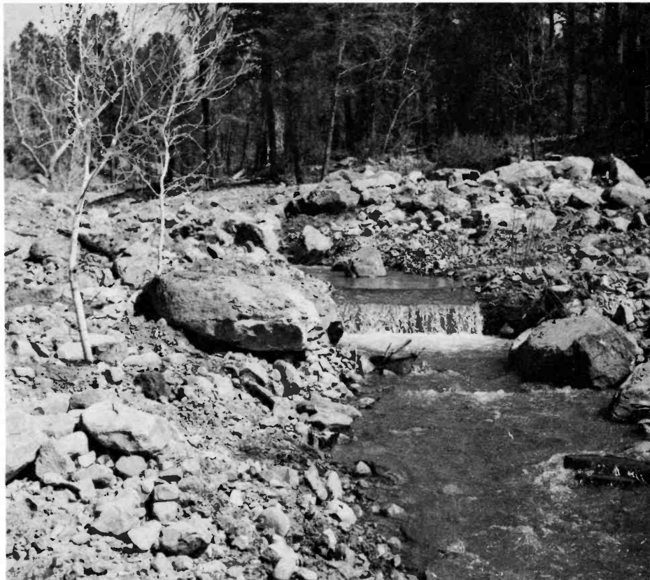
FIGURE 11. A REACH ALONG TONTO CREEK AFTER CLEAN-UP SHOWING PLANTED COTTONWOODS AND ARTIFICIAL POOL (COURTESY USDA FOREST SERVICE).
