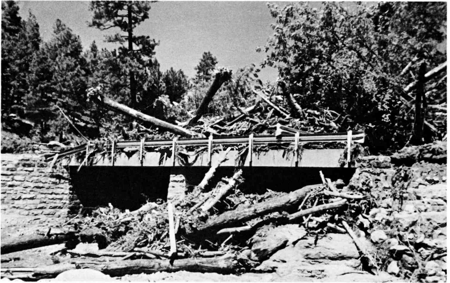
FIGURE 14. VIEW OF DOWNSTREAM FACE OF TONTO CREEK-HORTON CREEK BRIDGE AFTER THE 1970 LABOR DAY FLOOD. SEVERAL LIVES WERE LOST AT THIS LOCATION. (COURTESY USDA FOREST SERVICE).
