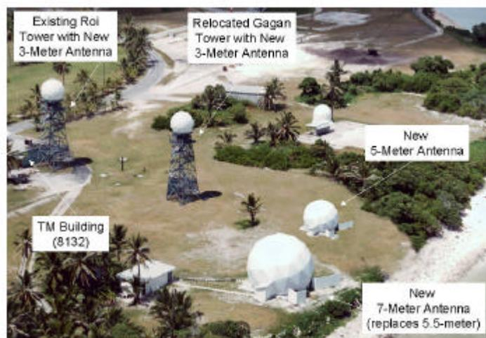
Figure 3. Final Roi-Namur Telemetry Antenna Configuration
