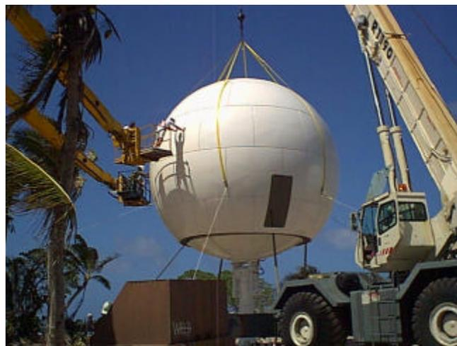
Figure 5. Installation of radome over new 5-meter antenna on Roi-Namur
