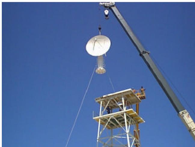
Figure 4. Installation of new 3.1-meter antenna on Roi-Namur
