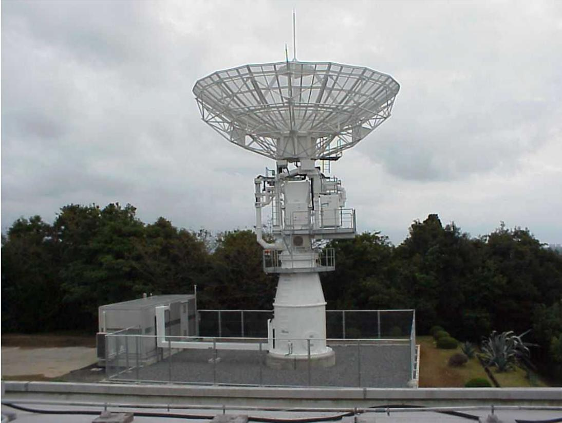
**Figure 3. Ground Station (New GN): 10m Tracking Antenna with Electronics Shelter at Left**
