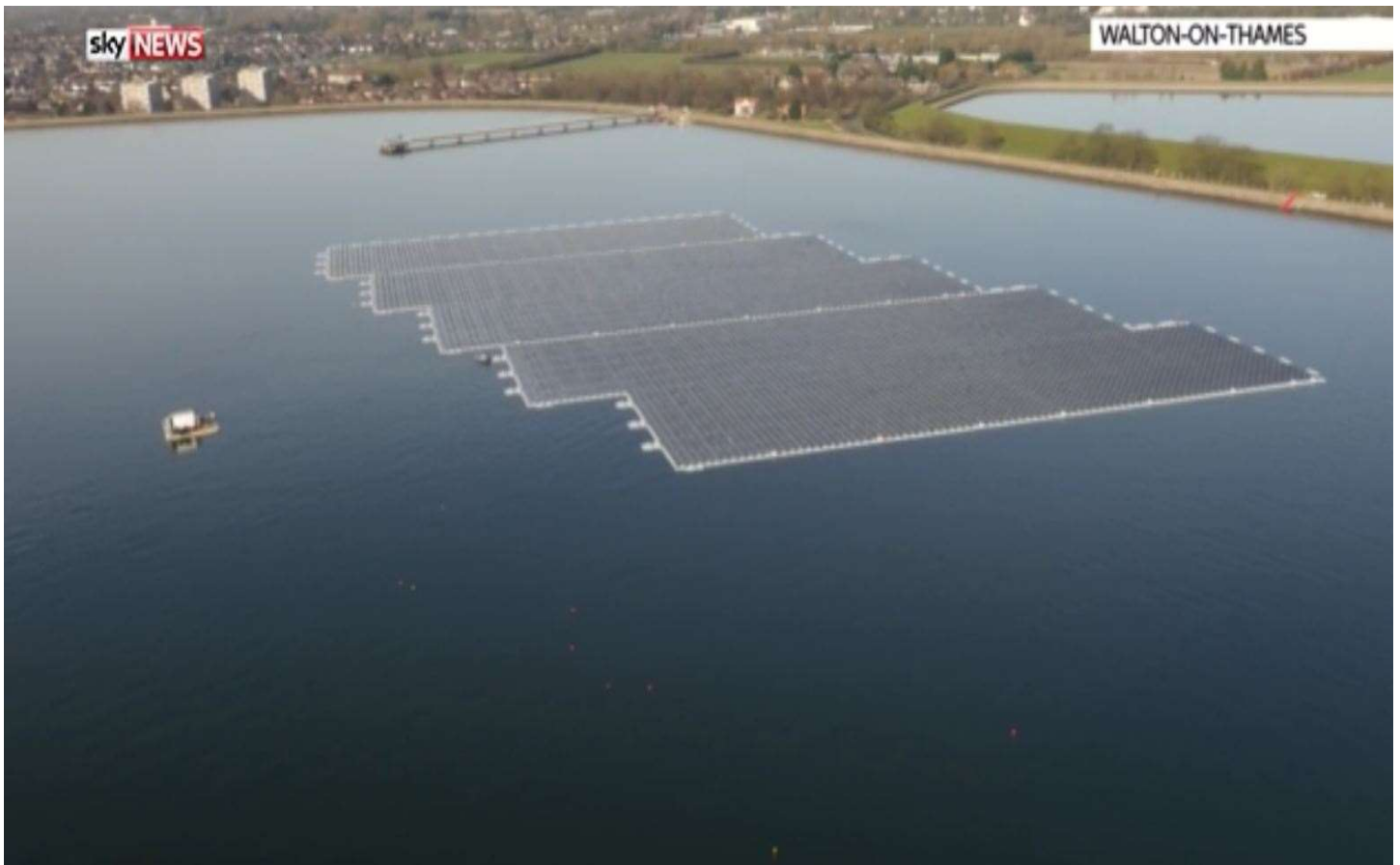
Figure 2QEII Reservoir, LightSource UK. Image courtesy of Sky News
