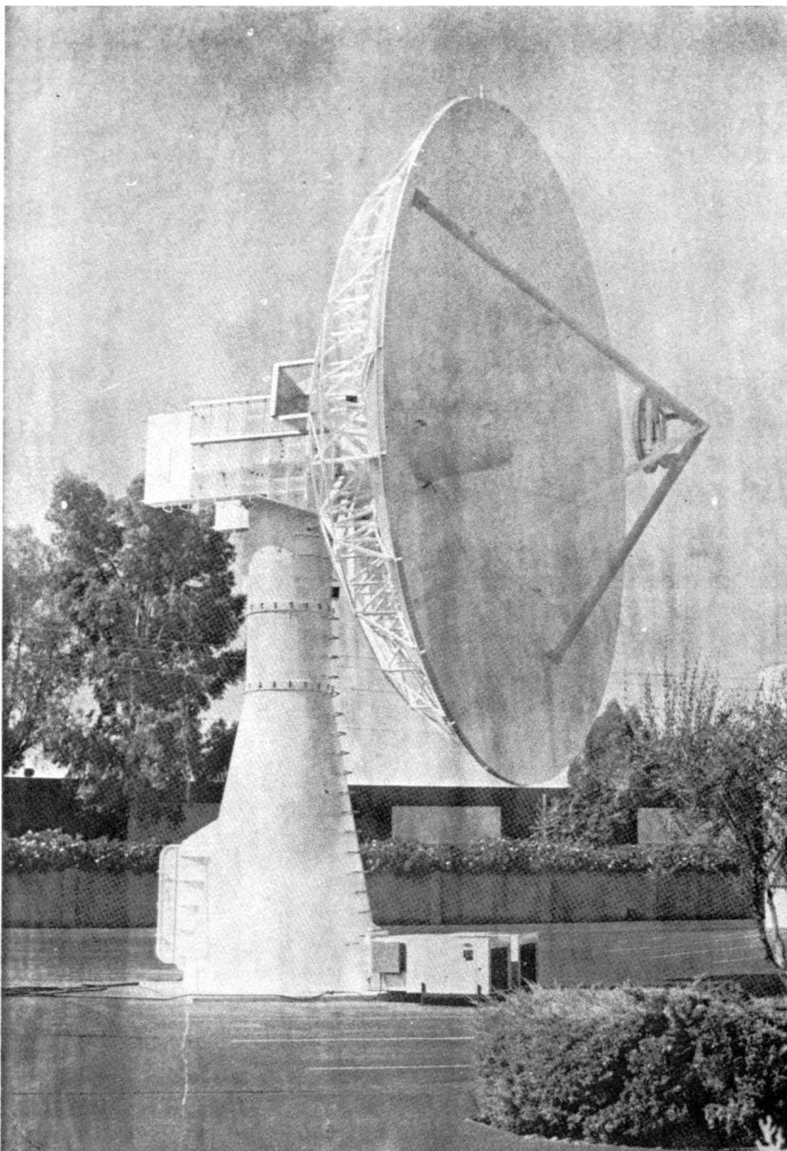
**Figure 3. Landsat Tracking and Receiving Antenna and Pedestal.**
